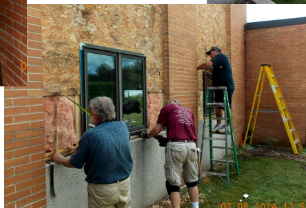
Removal of Styrofoam and installation of moisture block and other preparations.
